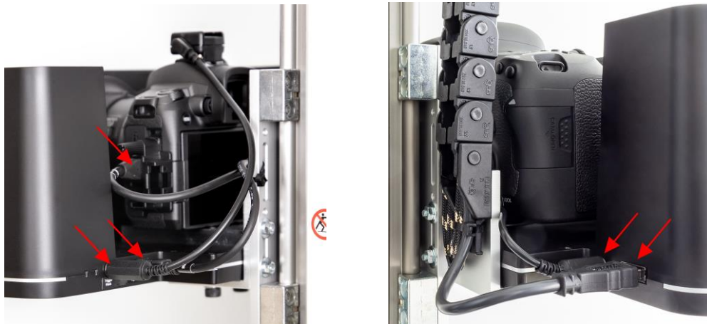
Fig. 12: Cable connections of PolFlash XE and camera to ATBM Tower (viewed from the left and right)
